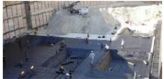
ENVIROMENTAL ATHORITY HEADQUARTER
